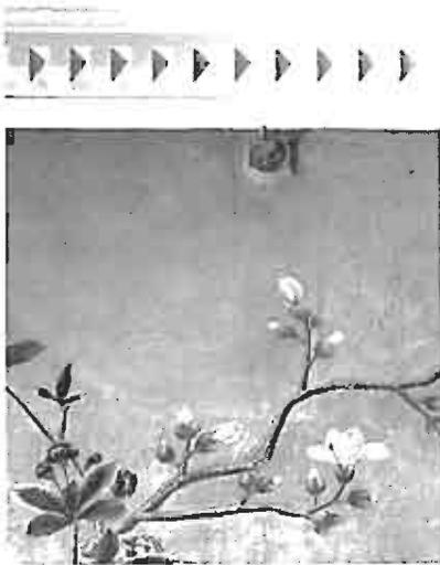
Figures 14 and 15 (above left and immediately above). In the Dillon Room at Blair House, Washington, DC, side-mounted sprinklers have escutcheons painted to match existing historic wallpaper.
